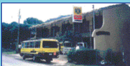
HOTEL - 15 well kept and clean rooms with all modern amenities while still keeping its beach ambiance. Pool, within 300 meters of the beach, 2 story construction with owners separate apartment. Hotel with good reputation in a good location. $575,000.
